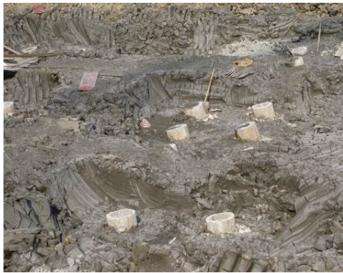
图 1 桩体倾斜图片展示 Fig.1 Photograph of inclined piles
