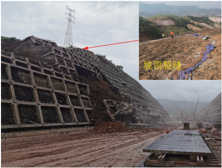
图 12 失稳挖方边坡概貌 Fig.12 Overall of an unstable excavated slope
